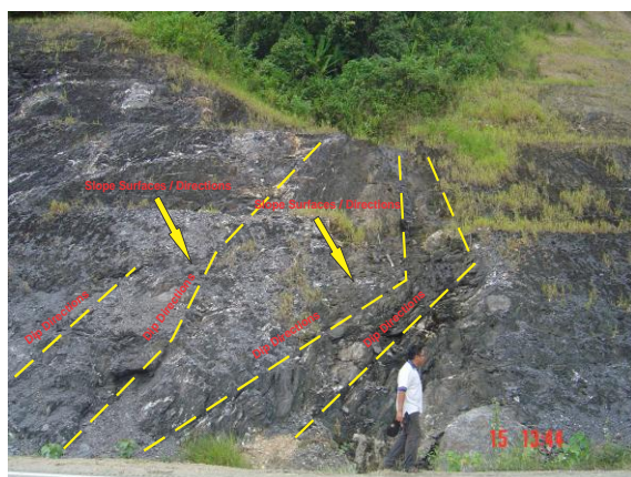
Figure 7. Slopes cut parallel to the strike and steeper than the dip of the day lighting planes then lead to landslide
