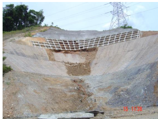
Figure 6. Damaged of slope physical state due to improper monitoring system
