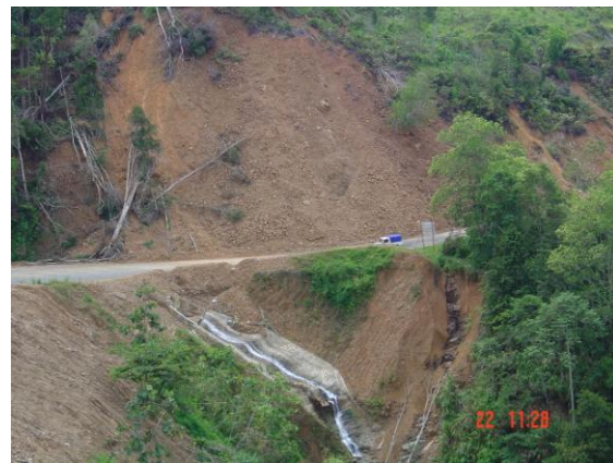
Figure 4. Photograph showing the settling soil block suffers from fracturing, stumping or flowing considerable lateral movement along the slip plane of the down slope (Location: KM 140 (S3))
