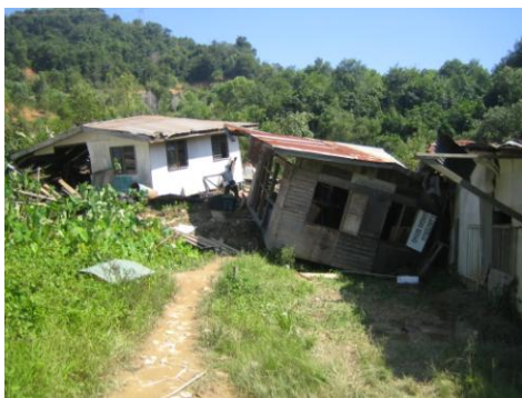
Figure 2. Photo showing the damaged house due to landslide hazard at Lok Bunuq village area (30th June 2006).
